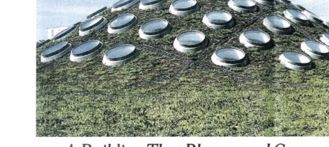
The new California Academy of Sciences is capped with a living roof that will be planted with native wildflowers and grasses.
